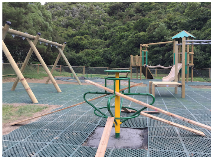
Upgrade at Brasenose Park nearing completion.
